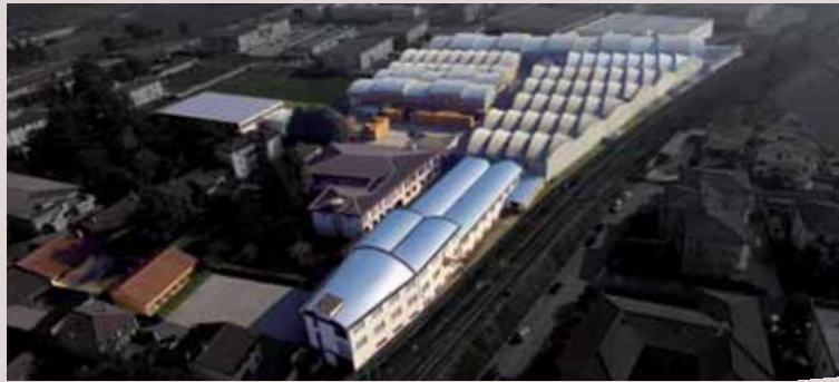
S•CAB sede/ headquarters - Coccaglio (BS) Italy
